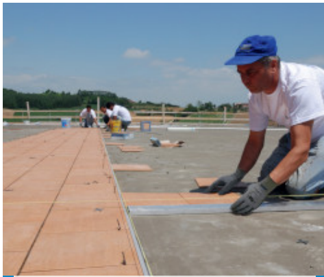
Installing ceramic with Kerabond + Isolastic
