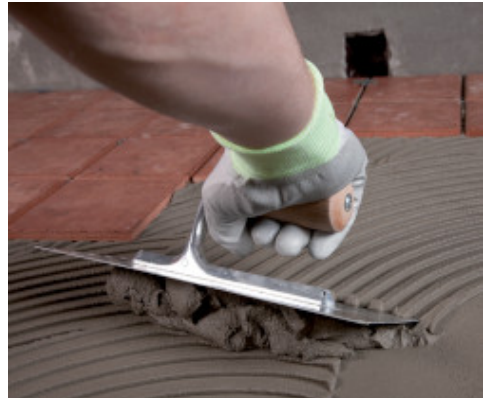
Laying Granirapid on a terrace waterproofed with Mapelastico Zero
