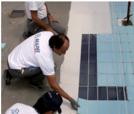
Laying ceramic tiles on Mapelastico Zero in a swimming pool
