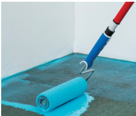
Second coat application of Mapeproof Primer
