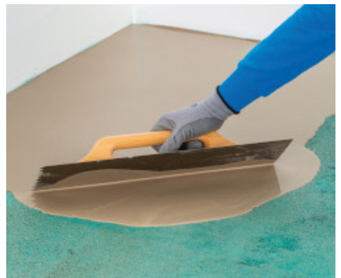
Self-levelling compound application on Mapeproof Primer
