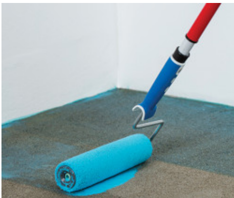
First coat application of Mapeproof Primer
