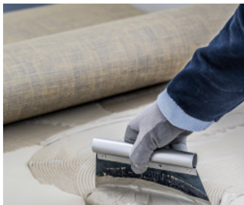
Application of Ultrabond Eco TX3 for installing linoleum
