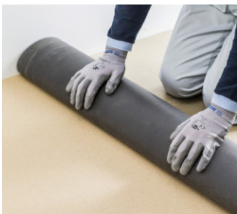
Acoustic underlay installation
