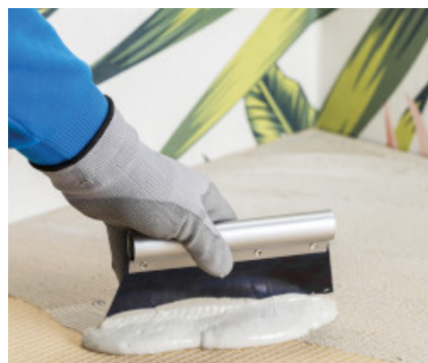
Ultrabond Eco TX3 application onto the acoustic underlay
