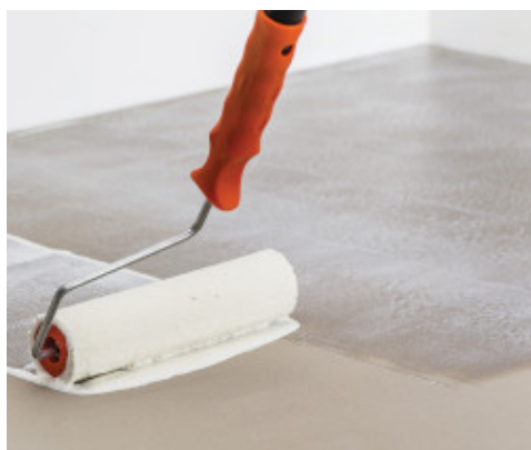
Ultrabond Eco TX3 application for fixing an acoustic underlay
