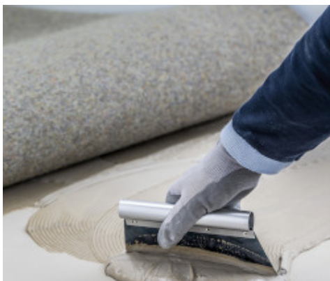
Application of Ultrabond Eco TX3 for installing needle-felt
